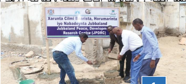
Upcoming Construction Prof. Gandhi (JPDRC) Centre
